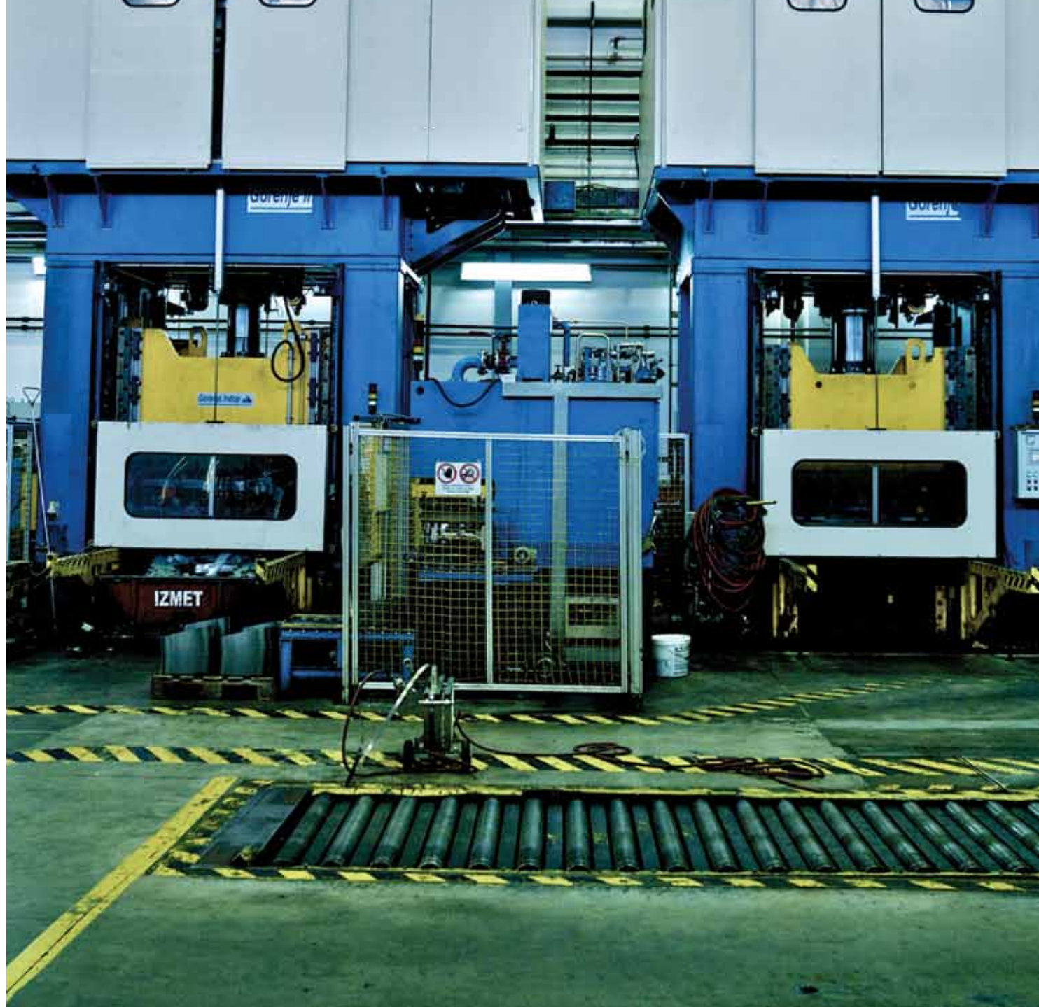
01 | PRESSES ON THE WASHING MACHINE LINE
