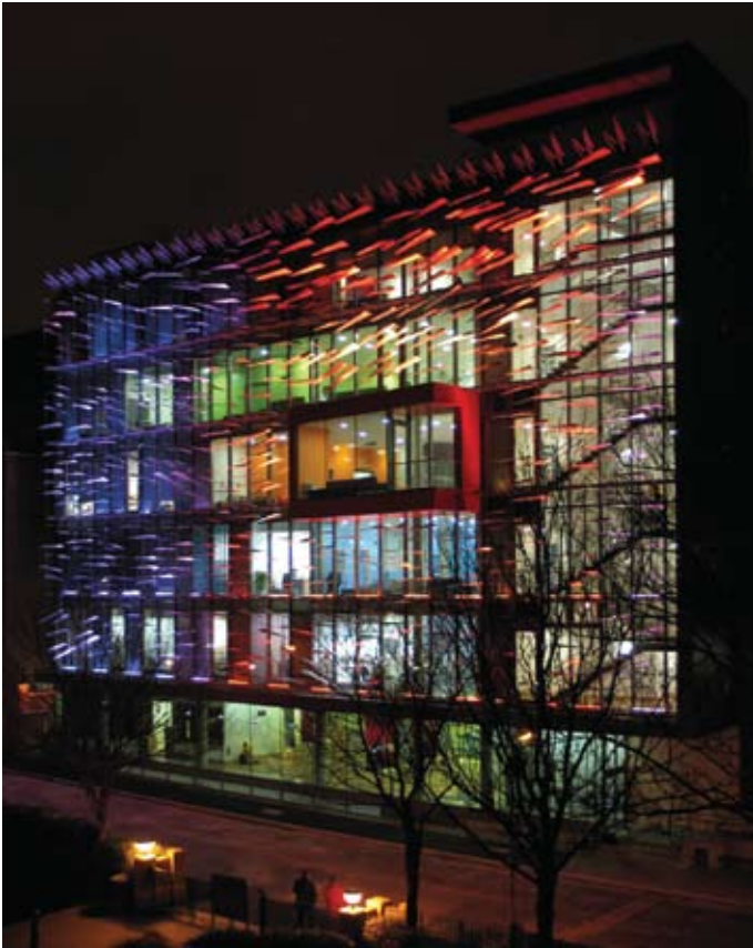
LED technology used to embellish the front of the Children's Eye Centre at Moorfields Eye Hospital, London, Great Britain
