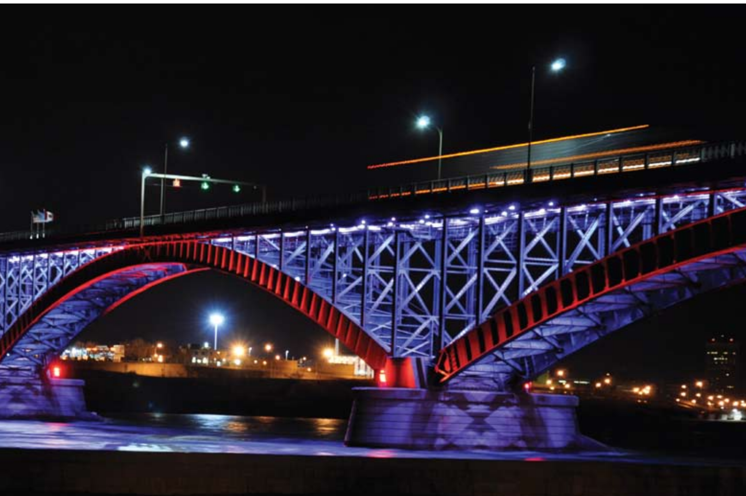
Peace Bridge over Niagara River, connecting Canada and USA, is illuminated by over 630 LEDs.
