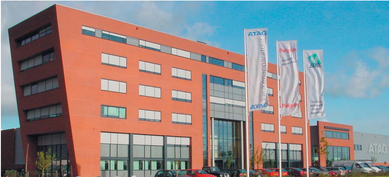
Headquarters : Duiven, the Netherlands
